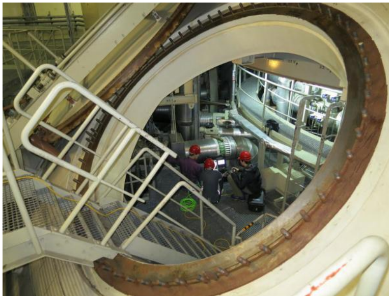
Figure 9: Deploying in the upper area of the reactor.
